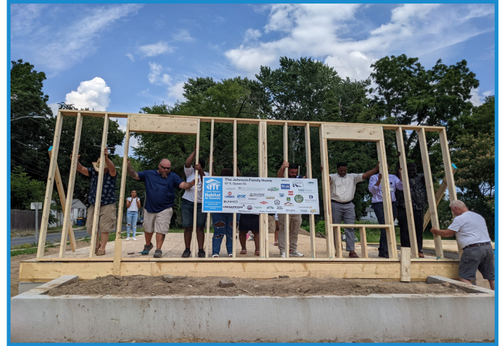
Habitat Wall Rasing
