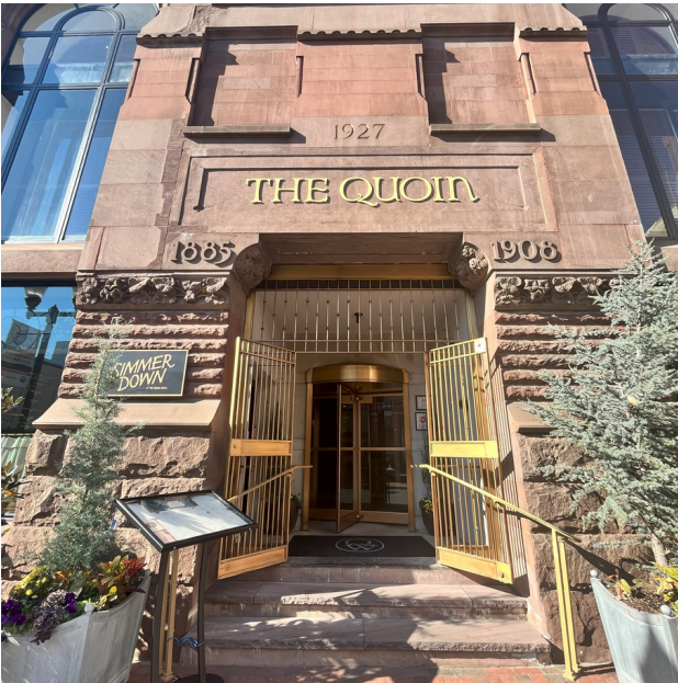
Large Project rehabilitation in Wilmington
