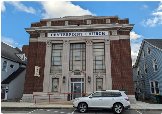
Rehabilitation of existing bank building
