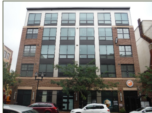
608 North Market Street BEFORE PICTURE OF SITE
