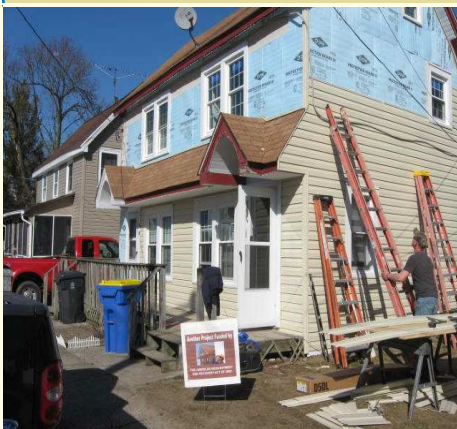
A Sussex County home receives rehab work through the CDBG-R program.
